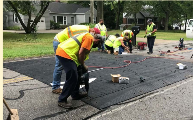
Source: City of Akron Location: Akron, OH
