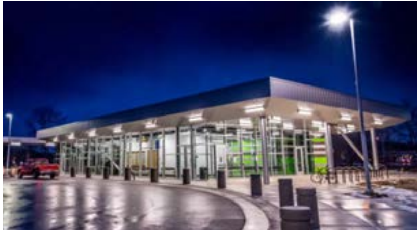
Image: East Lansing, MI Station, MDOT/Amtrak
